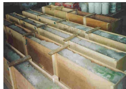
Fig. 5 Curing of rehabilitated beams with polymeric cement mortar
