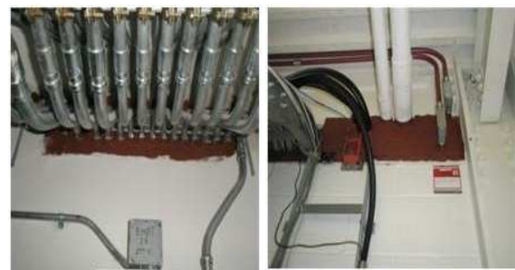
Fig. 9 Fire penetration protection system
