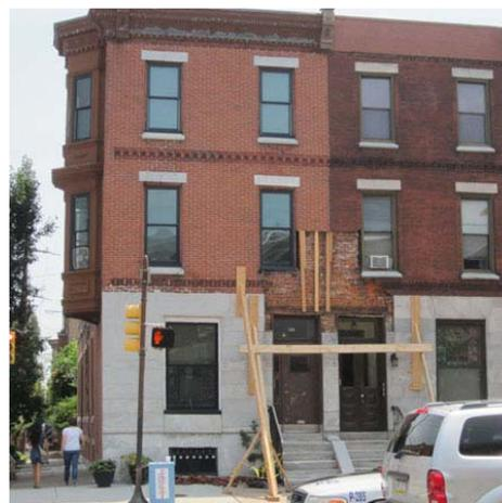
Fig. 1 Brick wall damage
