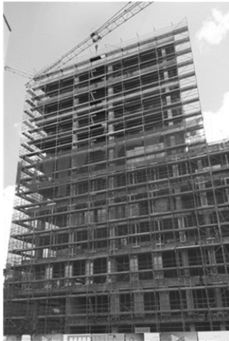
Fig. 1 A view of the scaffolding
