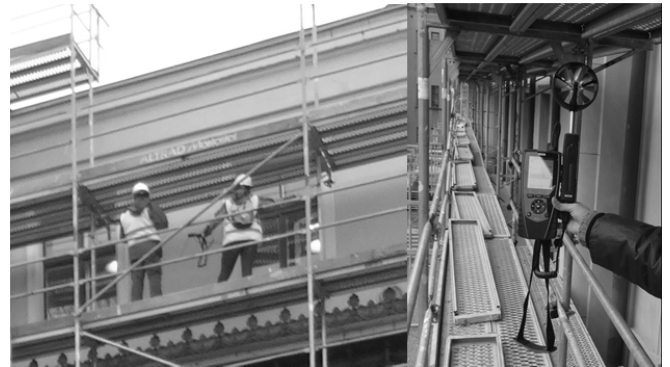
Fig. 3 The measurements on the scaffolding
