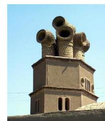
Fig. 6 Pipe Shape Wind-catchers
