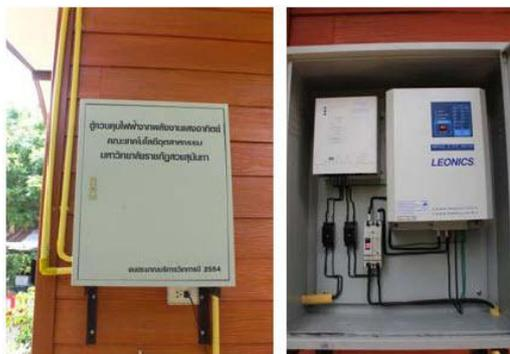
Fig. 3 Battery charge controller and AC distribution
